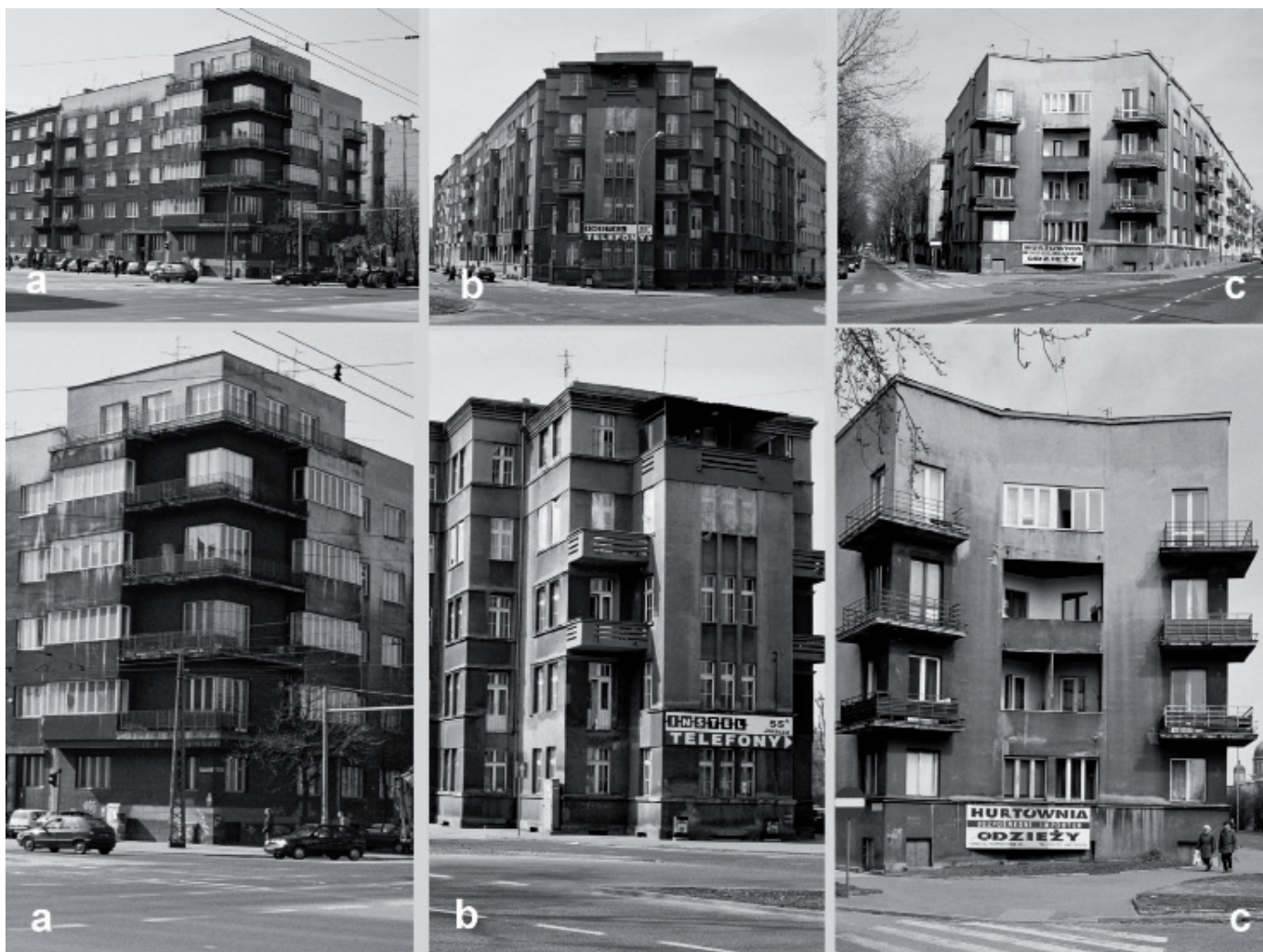
2. a. Corner tenement building in Łódź at 97 Kościuszki, the corner of Mickiewicza; b. Corner tenement in Łódź at 71 Jaracza the corner of Uniwersytecka; c. Corner tenement in Łódź at 36. Kamińskiego, the corner of Uniwersytecka. Photo by the author
