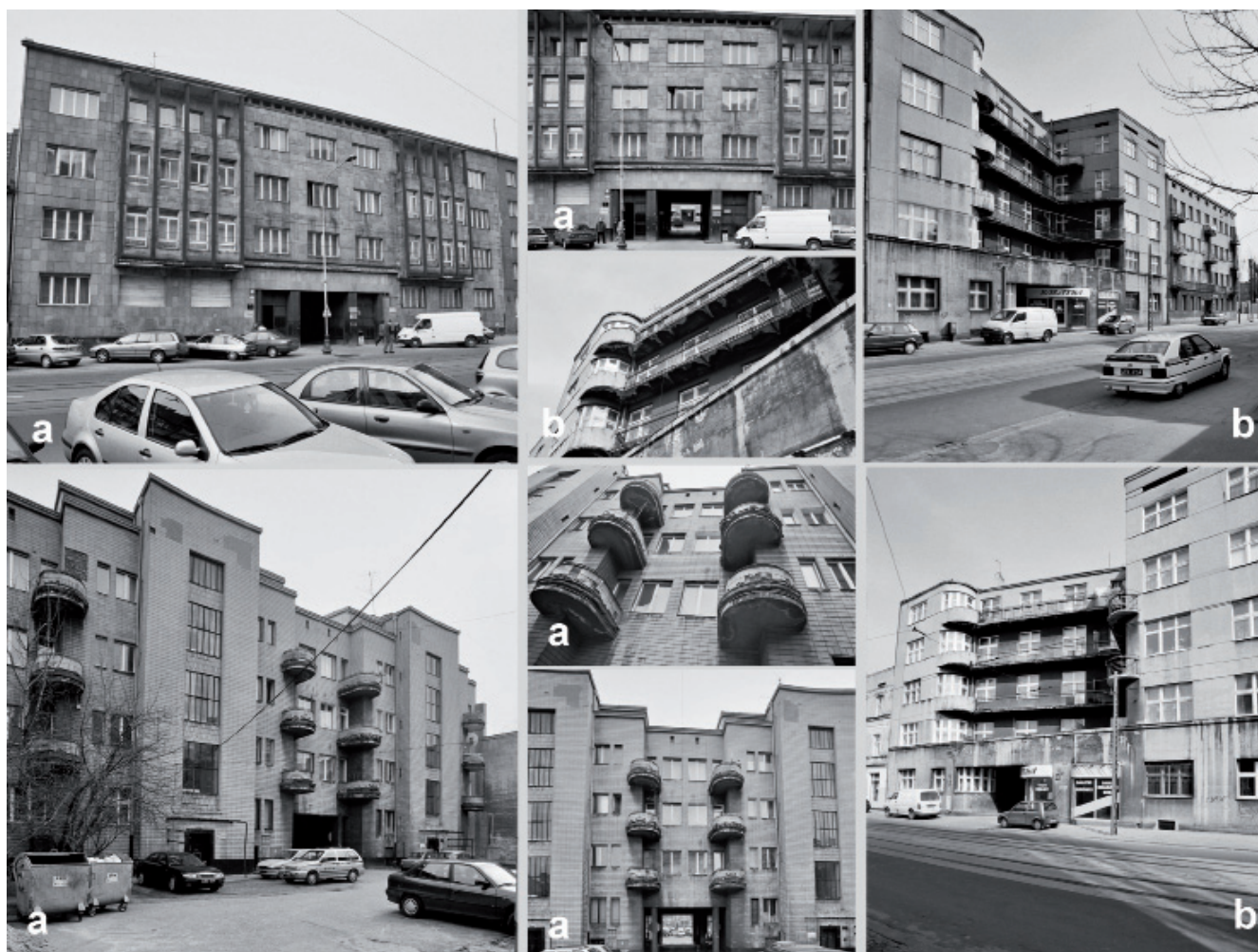
7. a. Frontage tenement in Łódź at 203/205 Piotrkowska; b. Frontage tenement in Łódź at 74 Gdańska. Photo by the author
