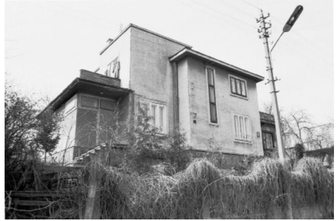
9. Villa in Grodno (10, Kirpiczna street, 1934); architect unknown. Photo by the author
