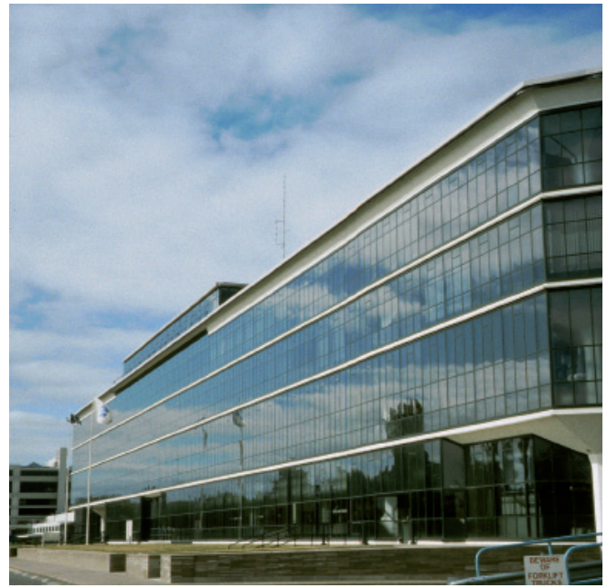
4. Boots D10 Factory, Nottingham, England, the new cladding system in 1996
