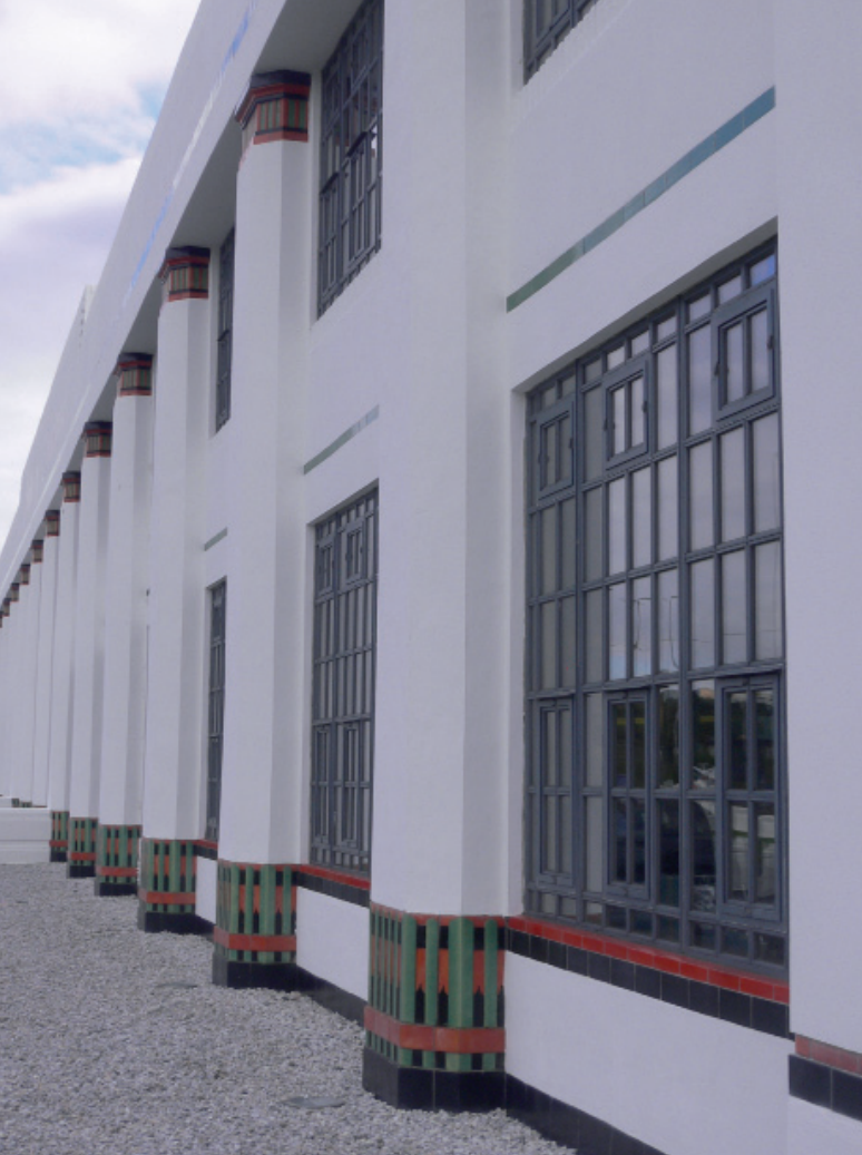
6. India of Inchinnan tyre factory 2007, by Wallis, Gilbert and Partners, 1929, after development by Graham Technology: windows adapted to carry extra panes of glass.
