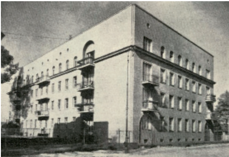
11. Warsaw, View of a house at 63, Filtrowa designed by Roman Feliński, ca. 1924.
