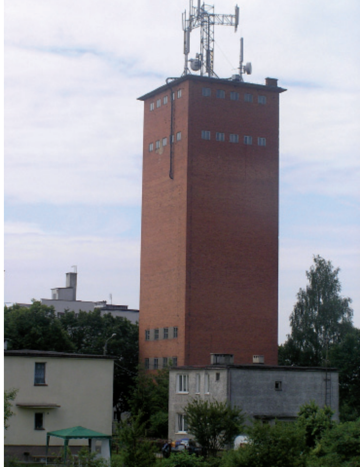
9. Morąg. Water tower, ca. 1928, designed by K. Frick; Photo by the author
