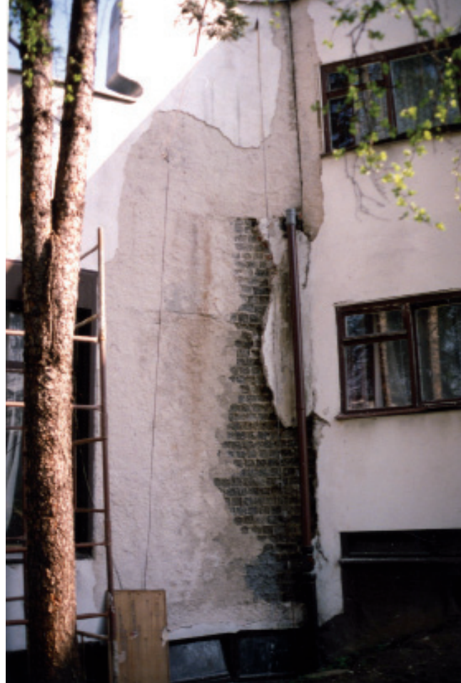
3. Wall damping between the left wing and the central part – 1993. Photo by the author
