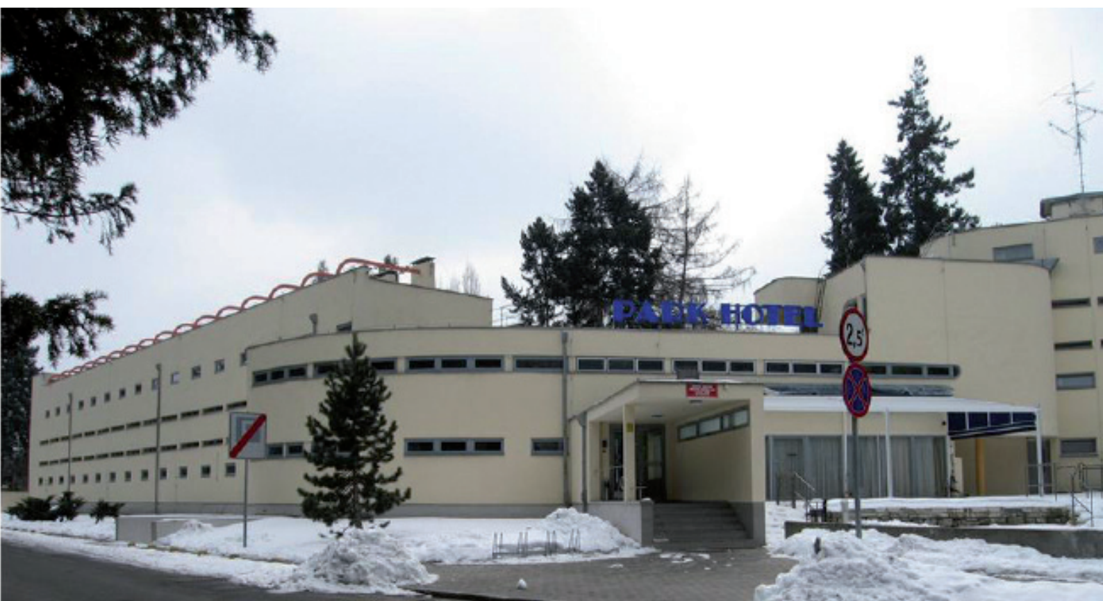
5. The building after elevations have been repaired, view from the street, 2005. Photo by B. Dubik
