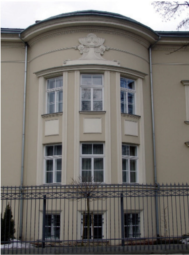
2. Tenement at the corner of streets Retoryka and Smoleńsk in Cracow, Wacław Krzyżanowski 1922, eastern elevation – the bay window. Photo by the author
