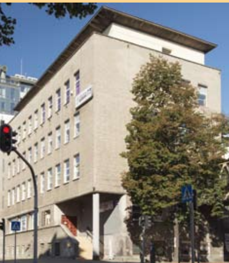
7. Budynek YMCA 7. YMCA building
