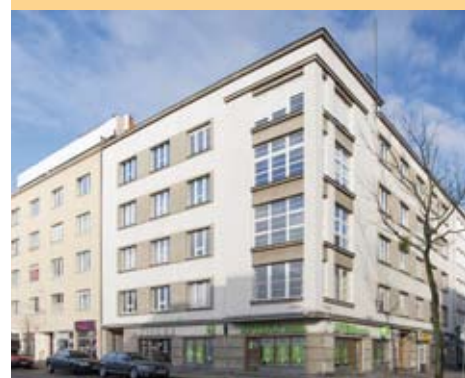
18. Kamienica Reicha i Birnbauma, ul. Abrahama, arch. E. Furschmied 18. Reich & Birnbaum apartment house Abrahama Street, arch. E. Furschmied
