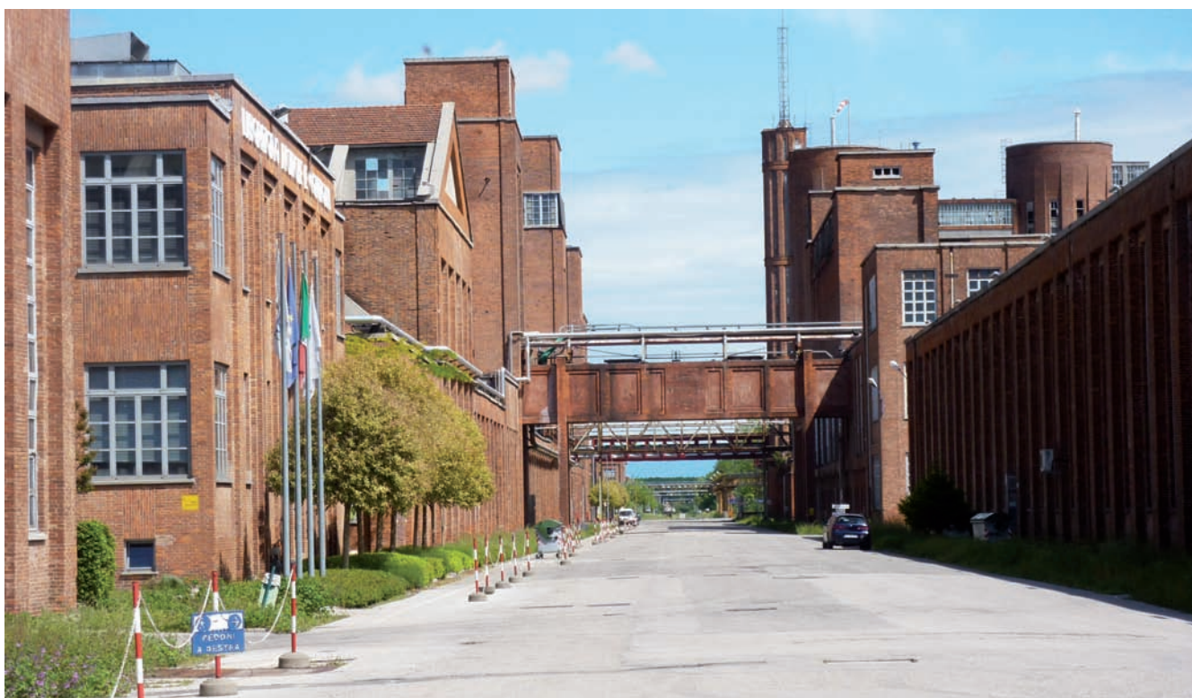
4. Torviscosa, architekt Giuseppe De Min, 1937 (fot. autor) 4. Torviscosa, architect Giuseppe De Min, 1937 (photo by author)
