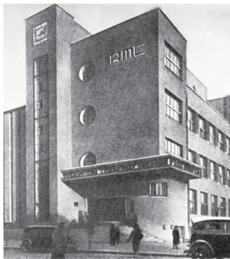
8. The building of an automatic telephone exchange, st. Freedom, 9, Kharkov, Frolov P., 1929-1930. (photo from A. Buryak's archive)
