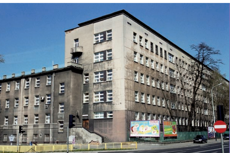
7. Gen. Felicjan Sławoj-Składkowski District Military Hospital, University Clinical Hospital Military Medical Academy - Central Veteran Hospital built in 1935-37 based on a design by: Stanisław Odynieć-Dobrowolski, Julian Lisicki, Janusz Krauss (photo: author)
